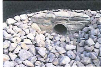
Armoured Swale Photo
