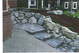
Boulder Retaining Wall Photo
