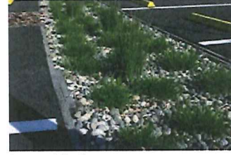
Armoured Swale Photo
